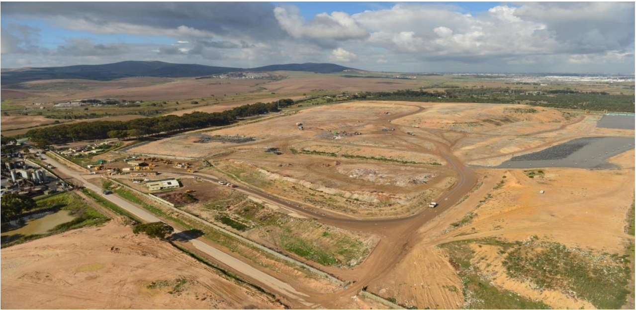
Figure 6: Visserhok (H: h) disposal facility
